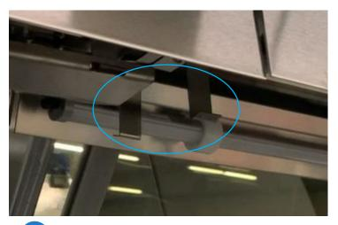
2 Locate the drip rail clips which are attached to the inside top of the display case and right in front of the light bulb. There should be two sets of brackets with one set on each end of the drip rail.
