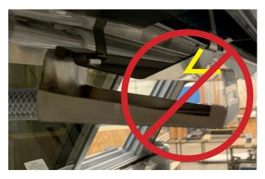
The front and back of the clip must be slid on over the drip rail. The V shape on the front of the catch pan did not get attached. Water will not drain properly.
